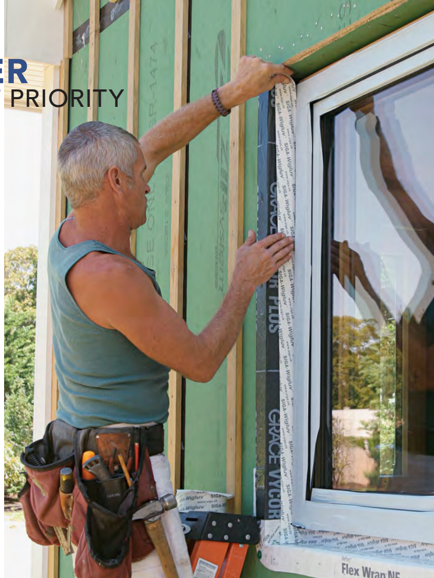
Multipronged approach. Modern flashing products more easily integrate windows and other penetrations with the WRB to keep water out, while vented rainscreens reduce pressure that can drive water into walls.
