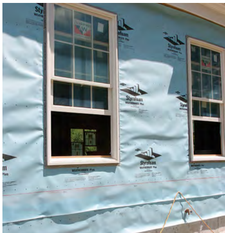
The trouble with housewrap. Despite long dominance as the go-to means of keeping a building dry, housewrap is widely regarded as a subpar choice for controlling air movement due to the difficulty in sealing seams, edges, and fastener penetrations.
